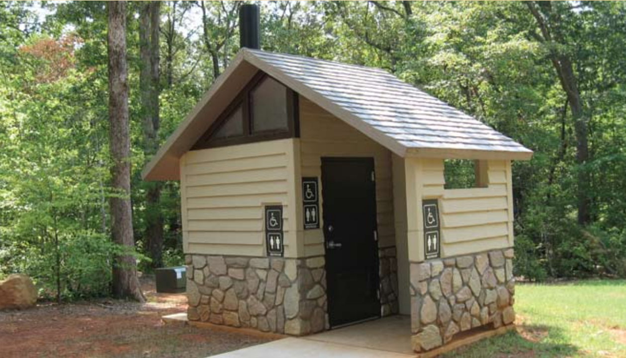
*Shown with Napa Valley rock and horizontal lap wall texture, and cedar shake roof texture.
